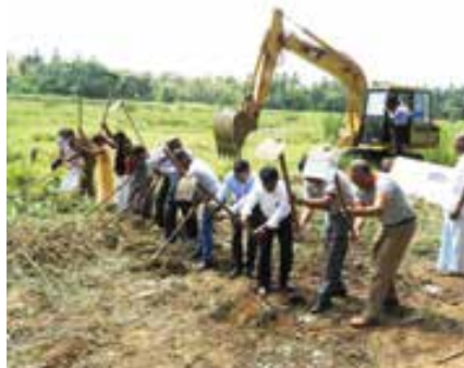
Commencement of restoration work
