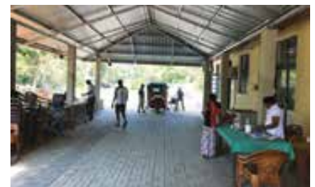
Newly-built covering hut at Elayapattuwa Divisional Hospital
